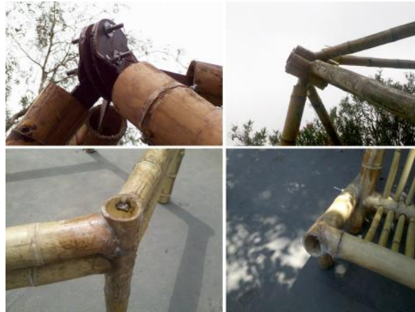
Figure 2: Junctions made by students from 2011 in the course Bamboo Technology.
